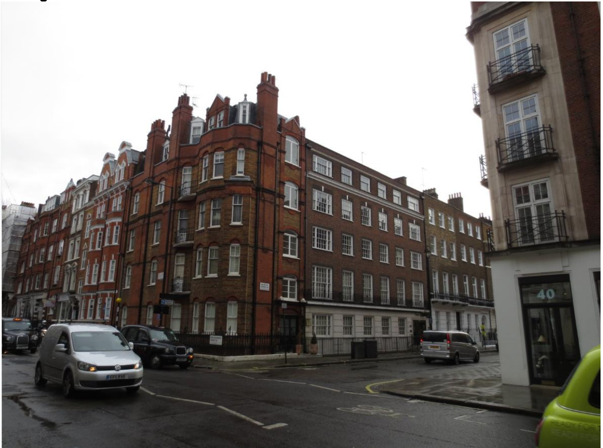
Existing front facade
